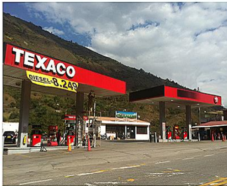
Texaco Gas Station Project in Colombia
